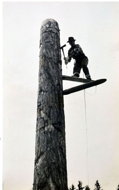
Old time springboard notches can still be seen in old stumps on the south end of Camano Island. In the earliest days Kyllonen said he didn't use safety equipment it was said as he climbed 125 feet and "pulled up a haulback block, hung it and threaded the line.
