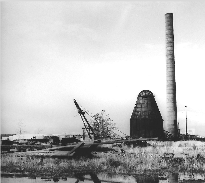
The photograph above shows the old style refuse/sawdust burner common in that era that stood next to the stack for years Accession No. 1987.04.27.40; Donor Photographer—Marion Duff
